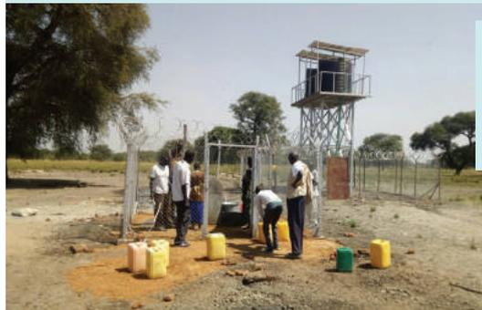
*Constructing small water distribution systems enables more people to access safe water in large village environments and reduces pressure on hand pumps.*
