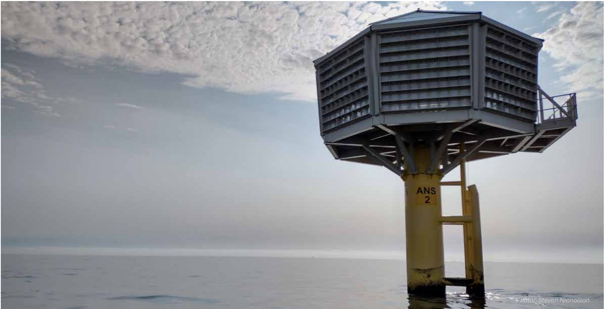
An ANS is an independent marine structure comprising of an octagonal topside with individual nesting spaces supported above the water on a single monopile. Each ANS has capacity for around 500 nesting spaces spread across eight rows of ledges per nesting face.
